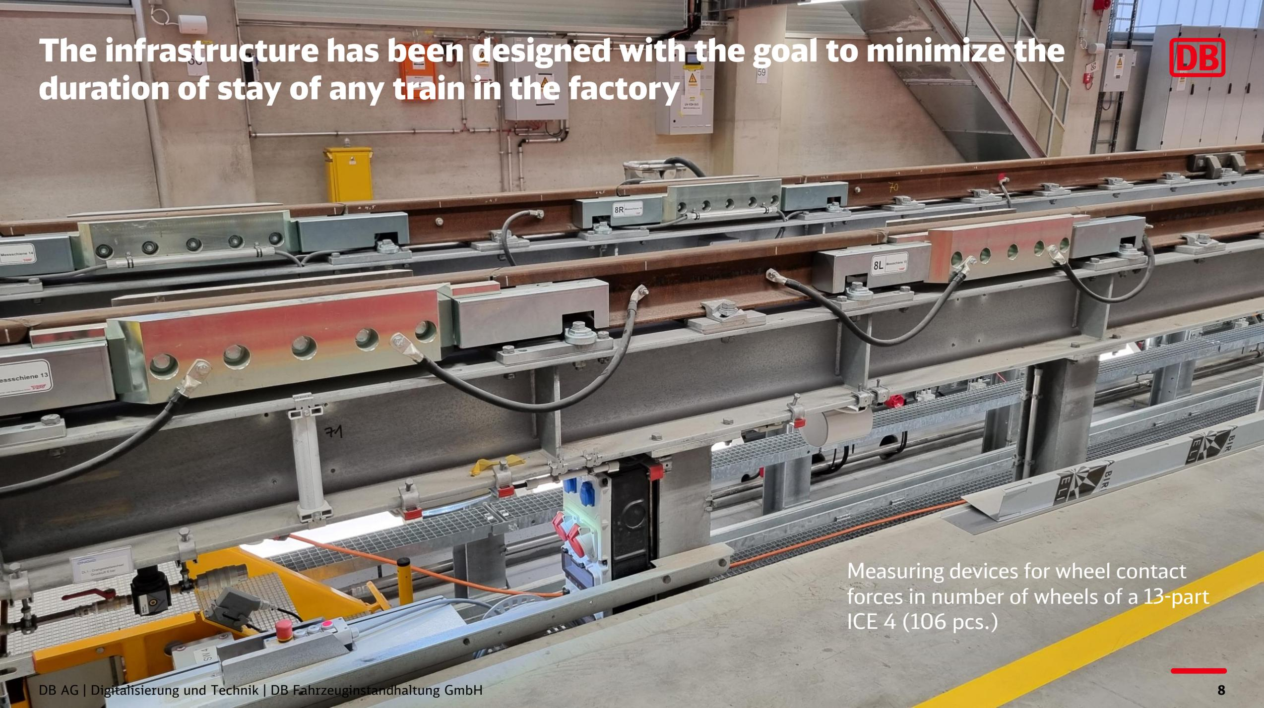
Measuring devices for wheel contact forces in number of wheels of a 13-part ICE 4 (106 pcs.)
