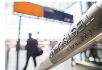
Braille handrail sign Railway stations
